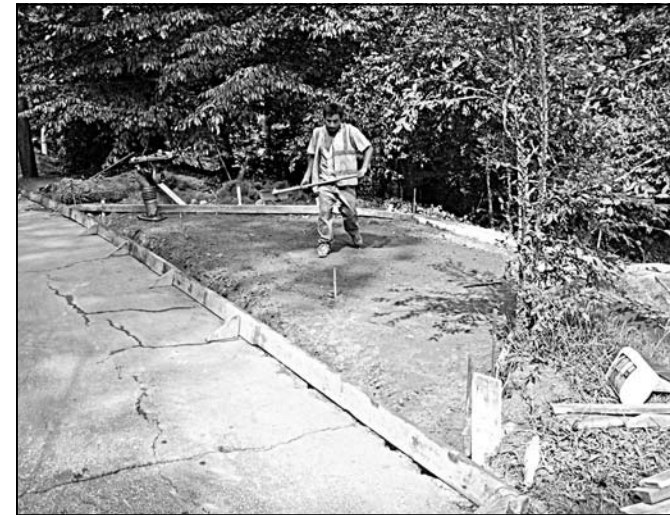
Worker on Land O'Lakes prepares a new driveway apron.
